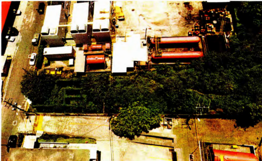
Site Location (in vegetated area) sandwiched between the two sections of the Fond Colé Power Plant
