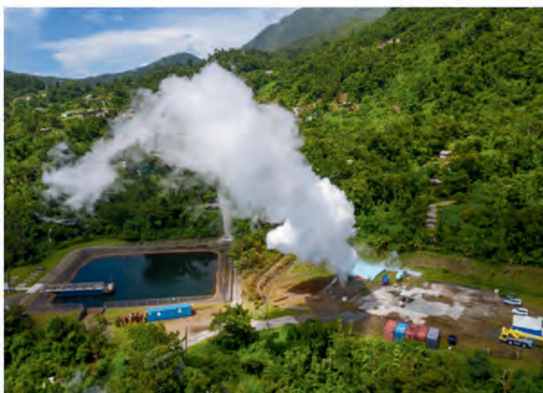
Geothermal Project Site. Photo credit: Nixon George/Quick Links Production via DGDC website.
